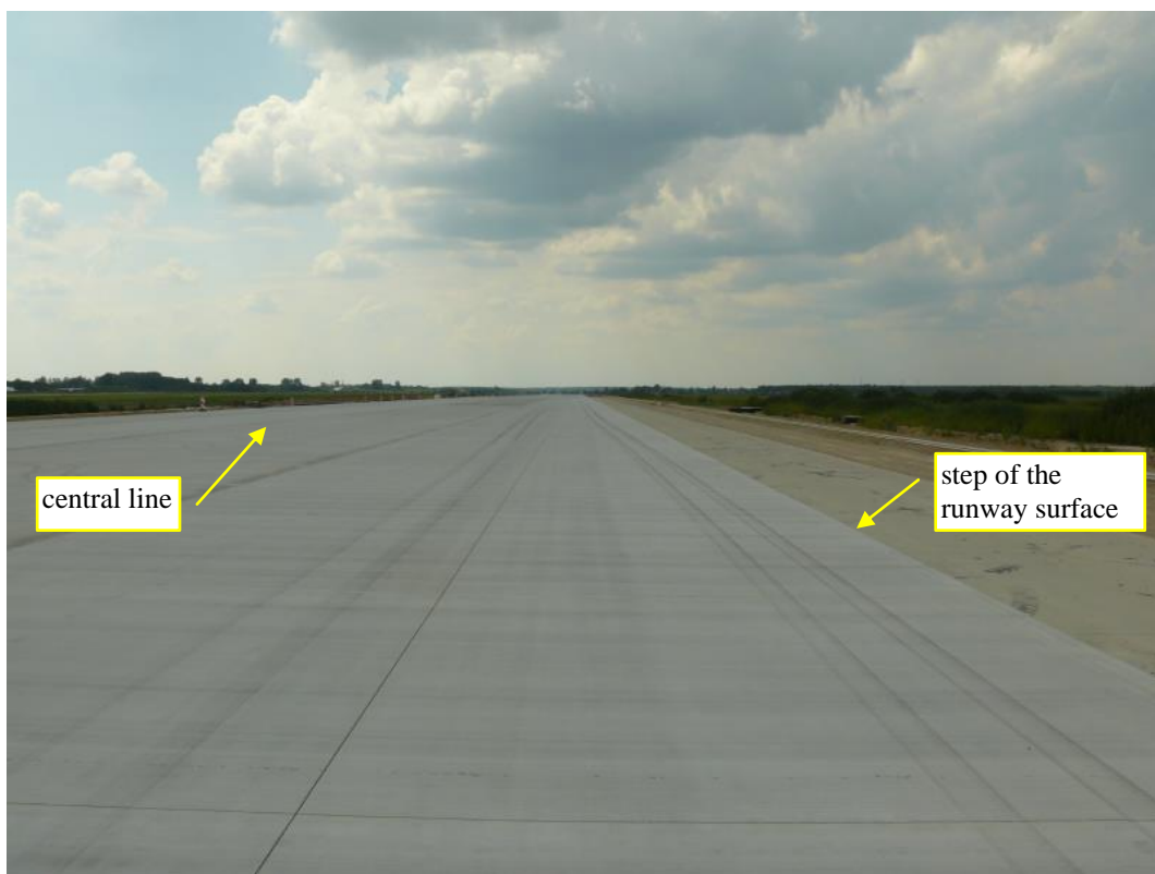
Photo 6. Tracks of the closest proximity between the airplane RMLG and the step of the newly constructed runway surface (1 m distance).
