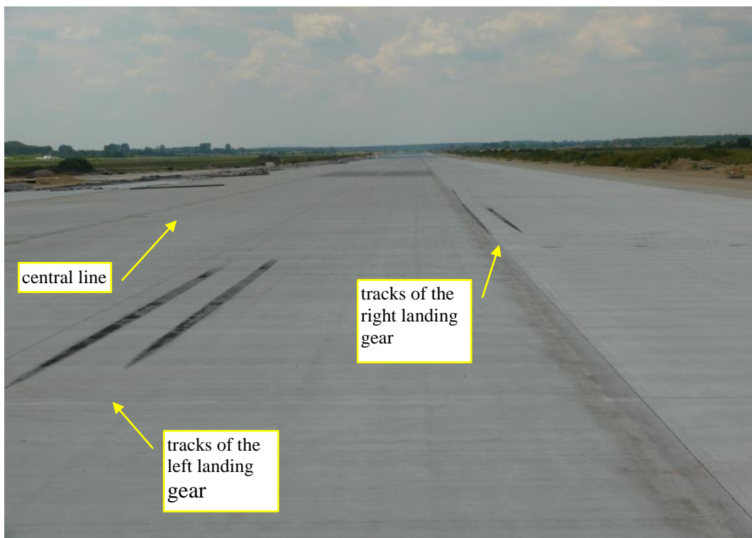
Photo 5. Touchdown tracks of the Bombardier CRJ-700 (~870 m from the beginning of the runway 27 surface).
