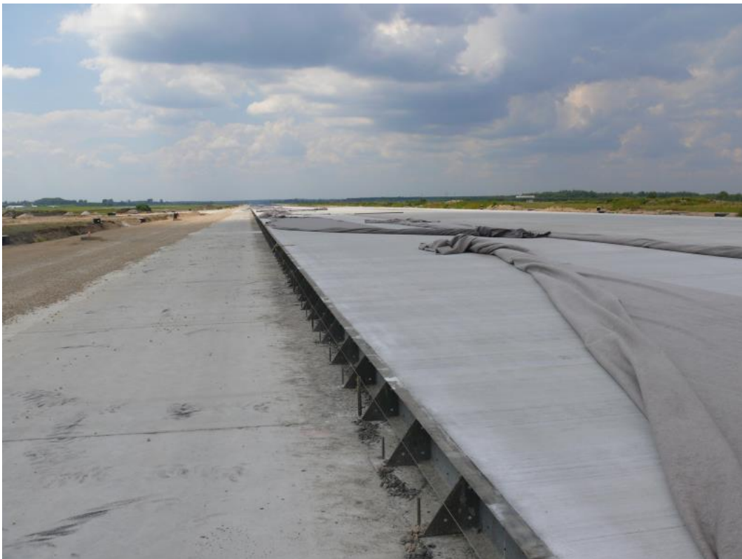
Photo 8. Structure forming/bounding the surface of the newly constructed runway (left side).
