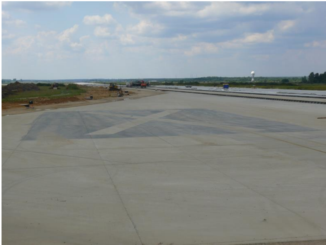
Photo 3. Marking of the closed runway under construction in the threshold 27 area.
