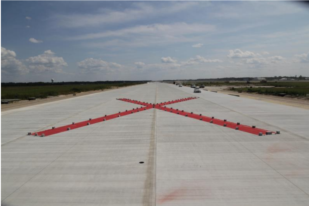
Photo 16. Marking of the closed runway under construction in the area of the threshold 09.
