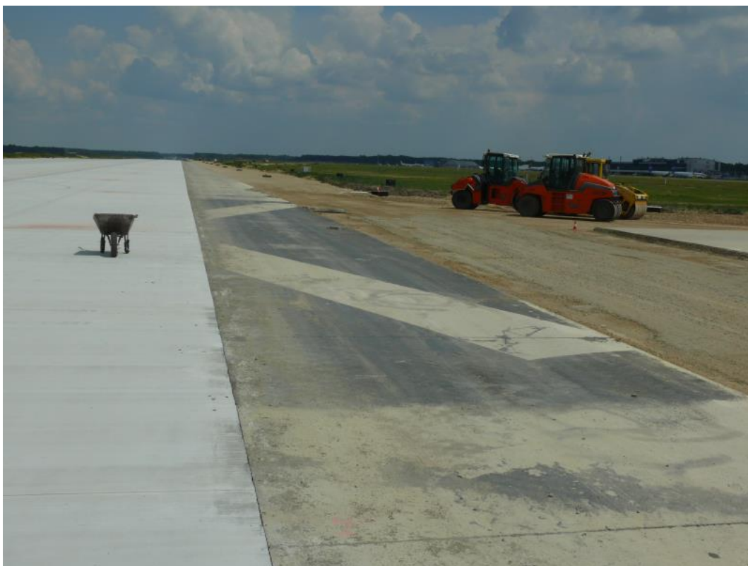
Photo 5. Marking of the closed runway under construction in the threshold 09 area partially covered with concrete.
