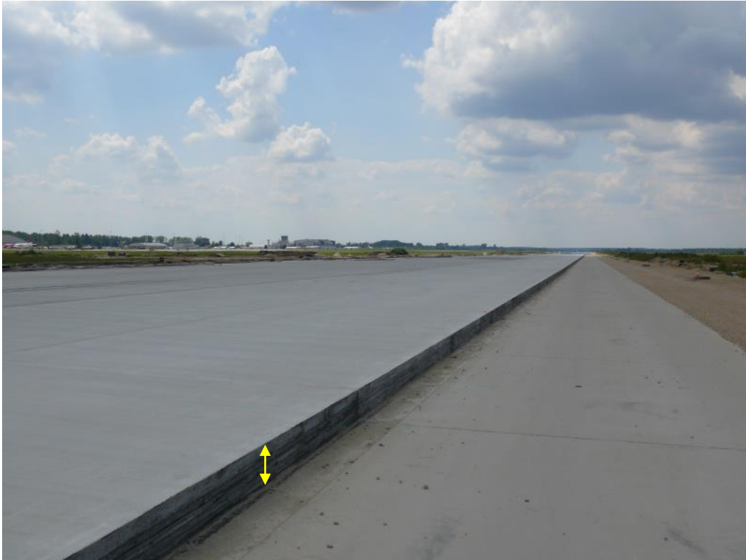
Photo 7. Step of the surface of the newly constructed runway (30 cm high – yellow arrow), right side.
