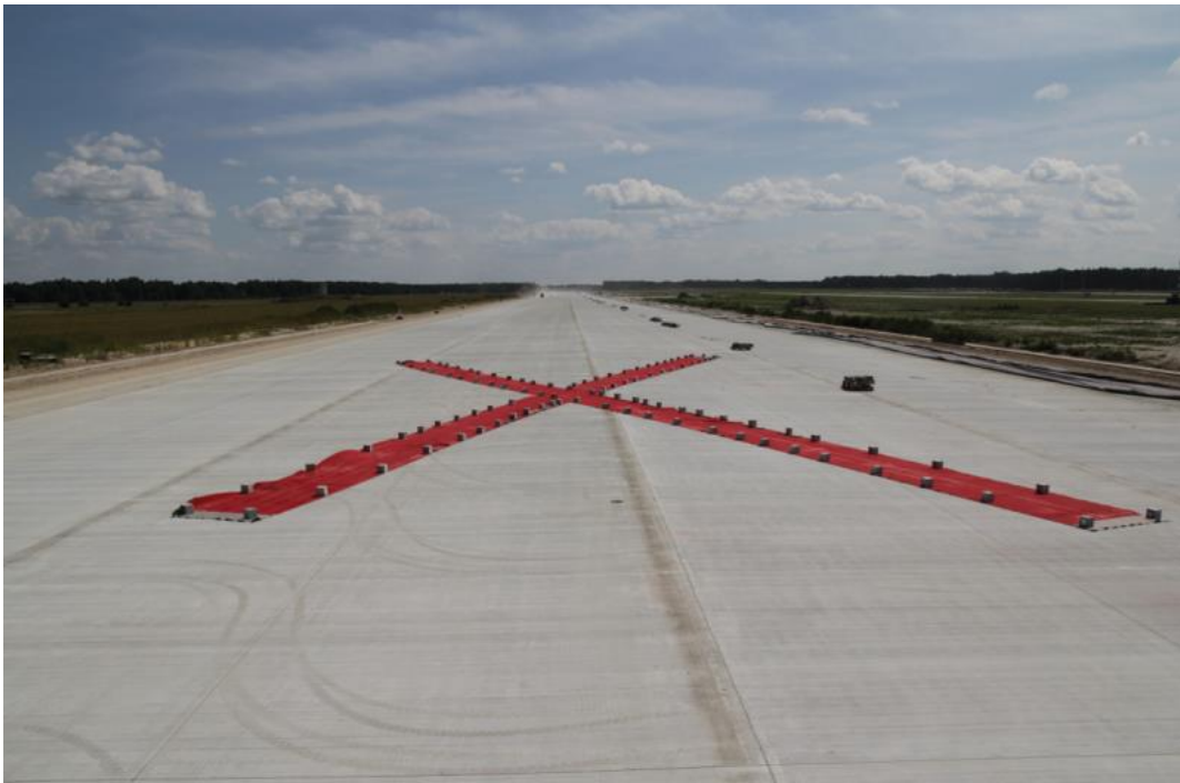
Photo 17. Marking in the middle of the closed runway under construction.
