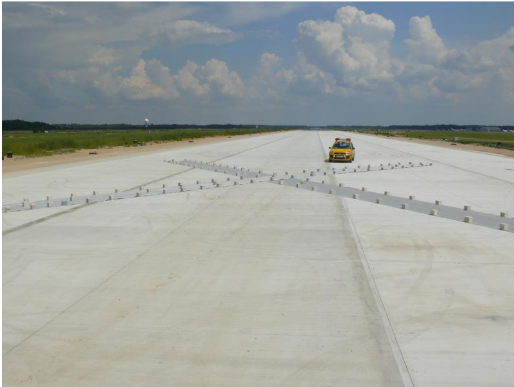
Photo 4. Marking of the closed runway under construction in the threshold 09 area.
