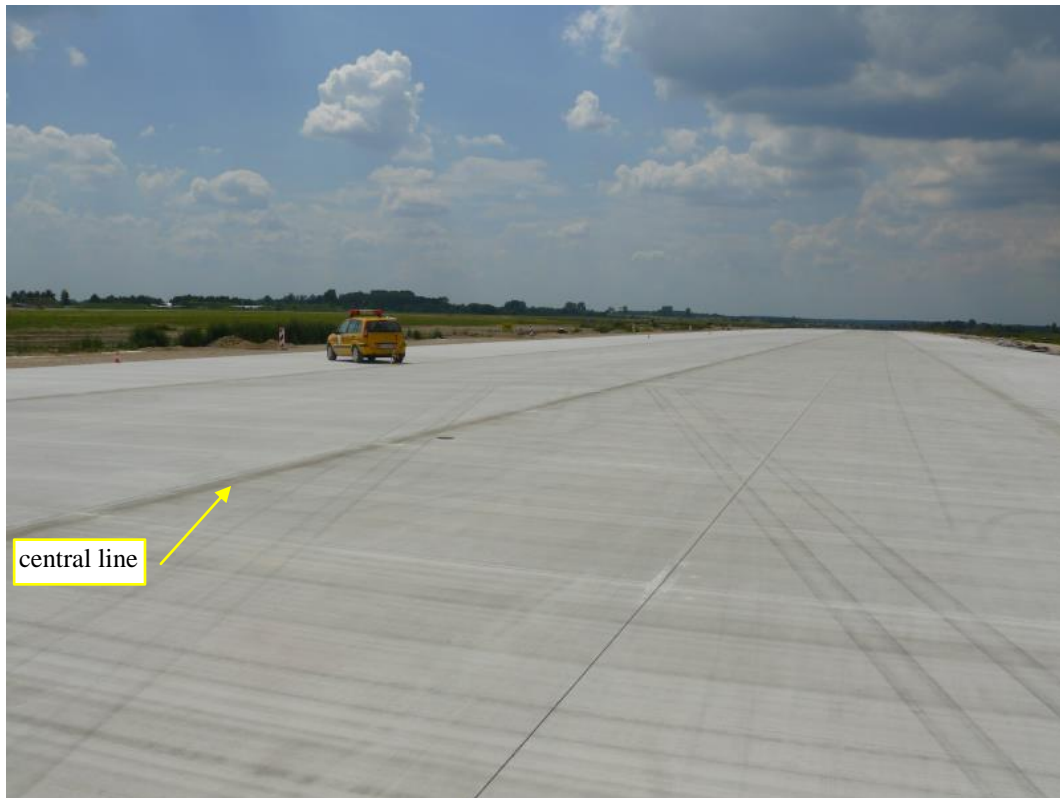
Photo 9. Tracks of the airplane stop on the runway under construction (~2700 m from the beginning of the runway 27 surface).
